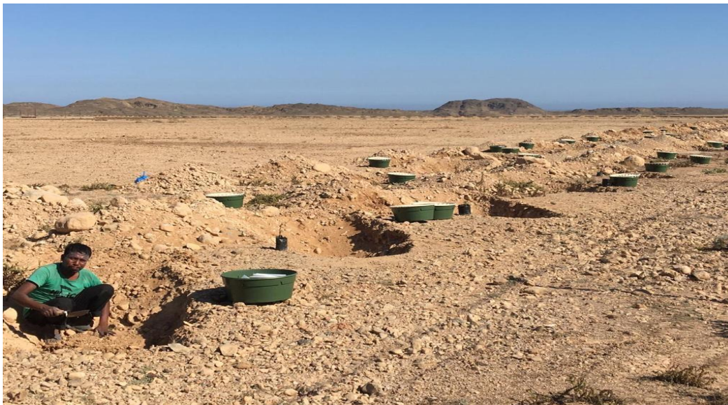
Photo of holes dug and wbx in place - plantation at Mirbat site, March 2019
